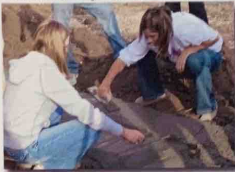
Amanda Schutz and Morgan Breinig smooth concrete for the greenhouse footings.
